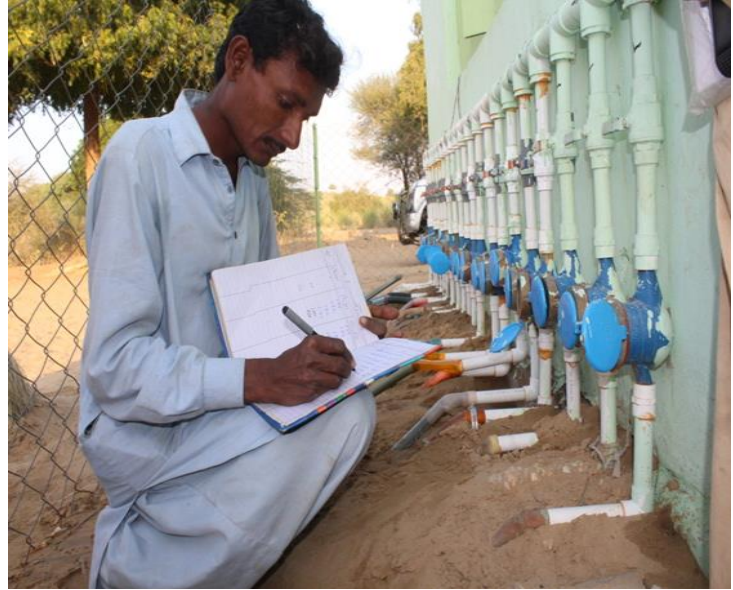
AWARE introduced meter system at pumps through these meters operator is measuring the quantity of water consumed by household
