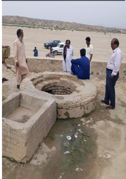
Fig 10 More than 100-year-old dug well in DG Khan Hill Torrents area gets water now when there is water in the waterway
